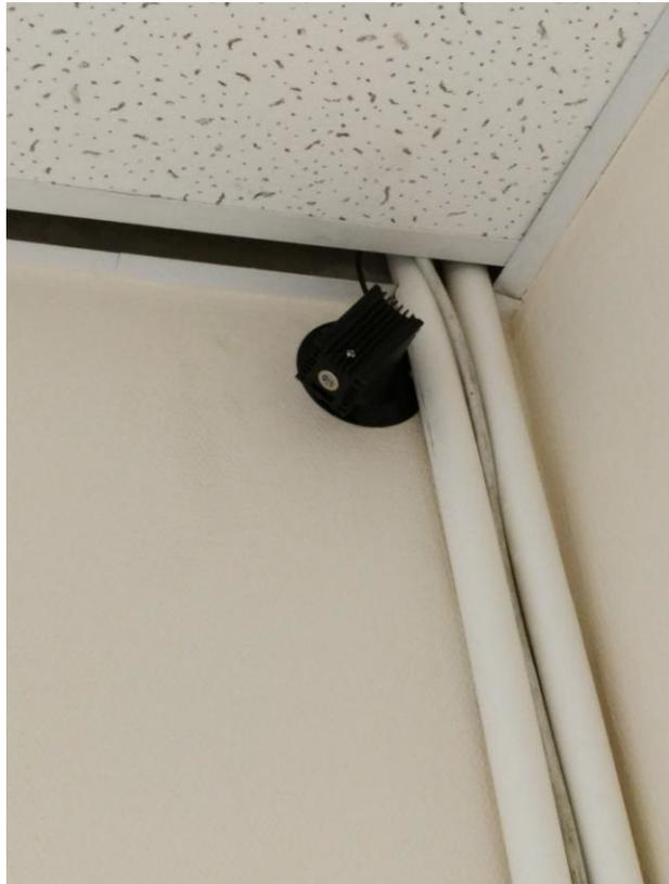
**Pic. 6 (Option 2) Mounting the infrared sensor on the wall**
